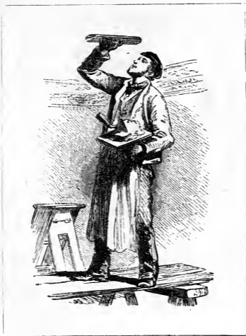
PUTTING UP THE CEILING.
